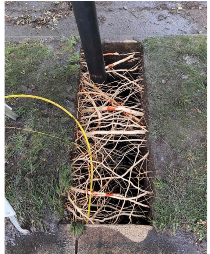
Our safe digging equipment can access underground utilities without damaging tree roots
